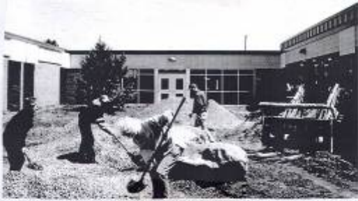
Initial groundwork and preparation.
